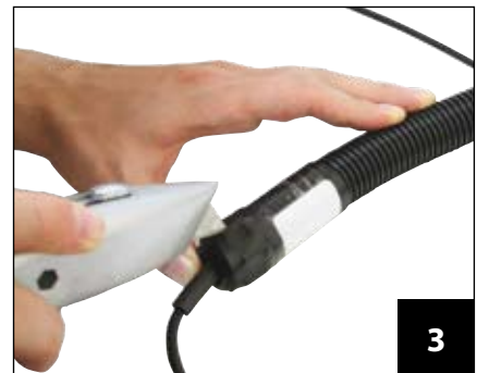
3 Cut the heatshrink that covers the gland.
